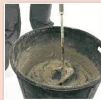
Mix only enough Porotherm bed joint mortar
