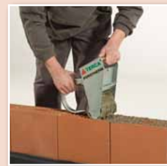
Apply using roller tool, scoop trowel or by dipping
