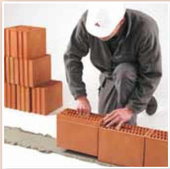
First course bedded in normal mortar
