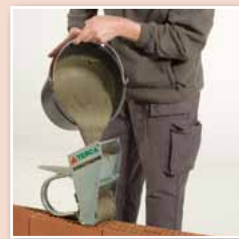
Apply using roller tool, scoop trowel or by dipping
