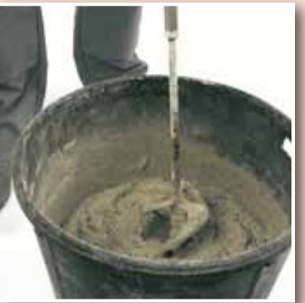
Mix only enough Porotherm bed joint mortar
